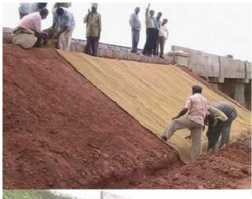
GAYATRI JUTE GEOTEXTILES for Embankment
